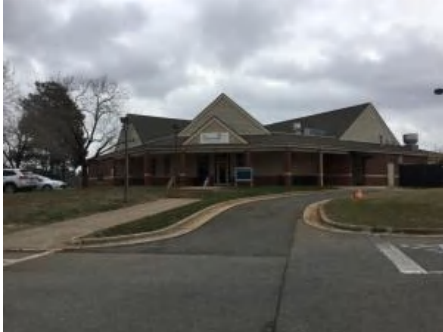
1). Southwest and Northwest Elevations - Feb 14, 2017
