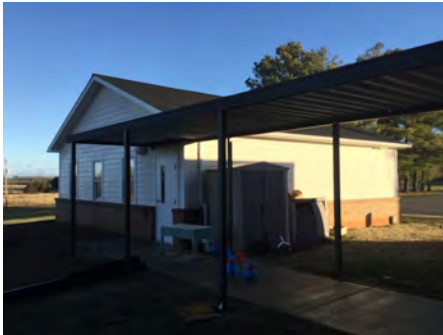
4). South Elevation - Feb 10, 2017
