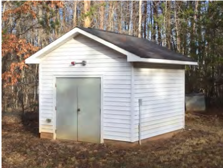
1). Southeast Elevation - Feb 10, 2017
