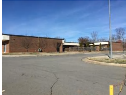
2). East Elevation - Feb 09, 2017
