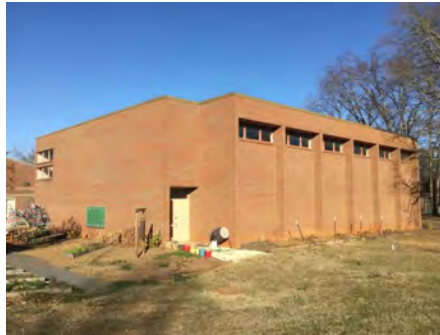
5). Southwest Elevation, Gym - Feb 10, 2017
