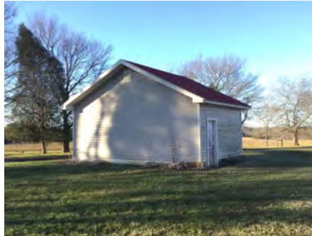
2). East Elevation - Feb 10, 2017
