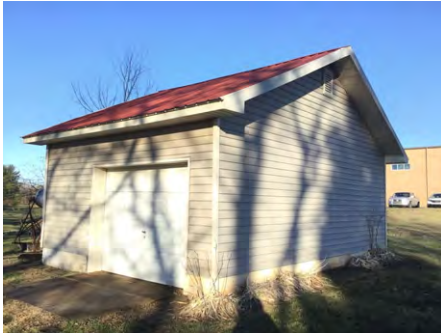
1). Southeast Elevation - Feb 10, 2017
