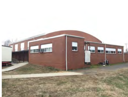
5). North Elevation - Jan 23, 2017
