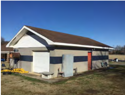
4). Southeast Elevation - Feb 10, 2017
