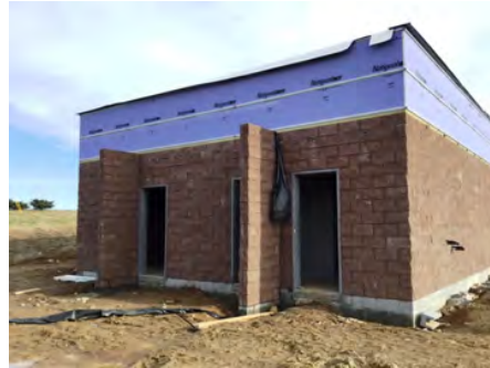
2). North Elevation - Jan 24, 2017
