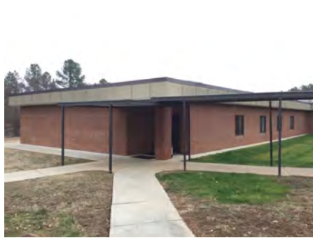
2). Southwest Elevation - Jan 23, 2017
