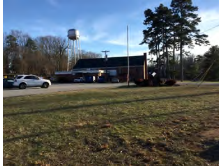
2). North Elevation - Feb 14, 2017
