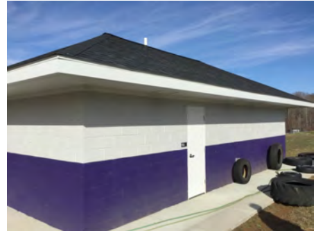
3). South Elevation - Feb 11, 2017
