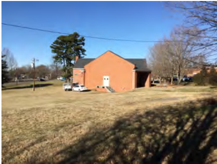
4). South Elevation - Feb 14, 2017
