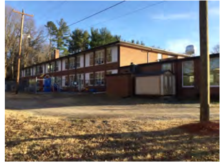
3). Northeast Elevation - Feb 14, 2017
