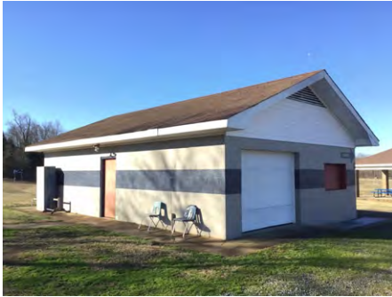
1). Northeast Elevation - Feb 10, 2017
