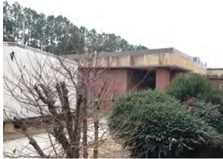
2). North Elevation - Jan 23, 2017
