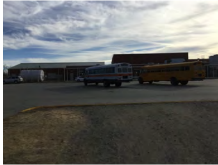
2). North Elevation - Feb 13, 2017
