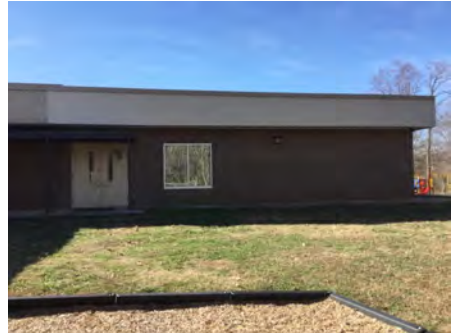
3). Northeast Elevation - Feb 13, 2017
