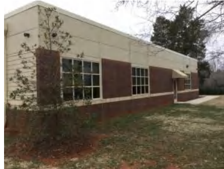
2). Northeast Elevation - Feb 14, 2017
