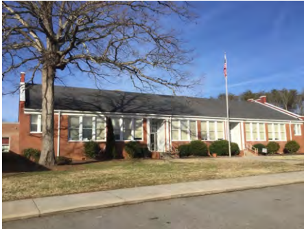
1). East Elevation, 1940 Bldg - Feb 10, 2017
