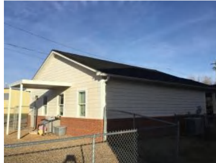
2). Southeast Elevation - Feb 10, 2017
