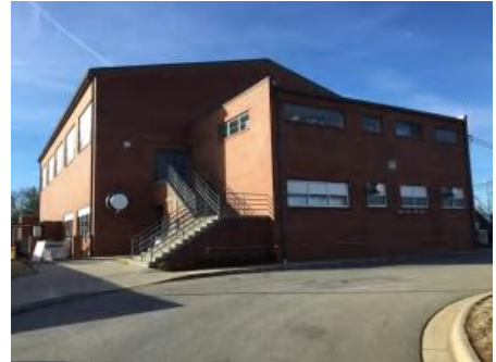
3). Northeast Elevation - Feb 09, 2017
