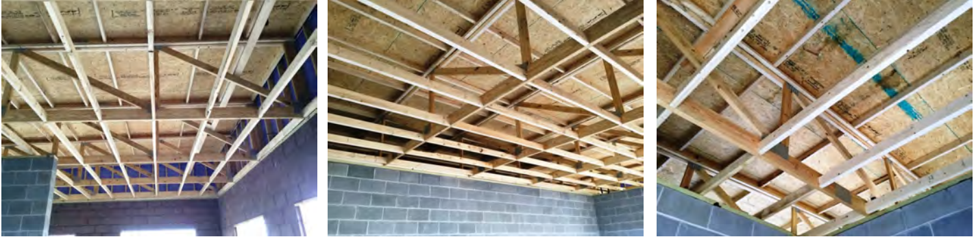
System: B1020 - Roof Construction
