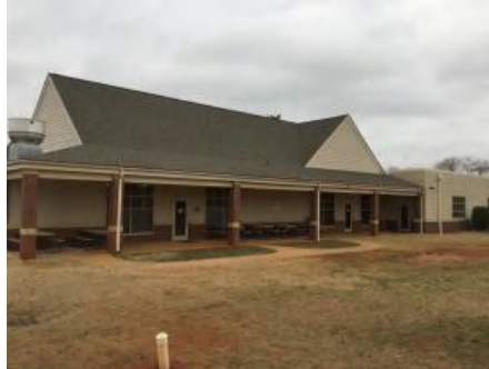
2). Southeast Elevation - Feb 14, 2017
