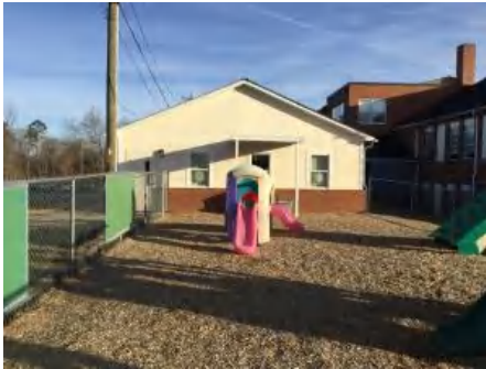
4). South Elevation - Feb 10, 2017
