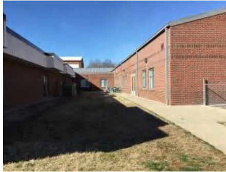
2). South Elevation - Feb 09, 2017
