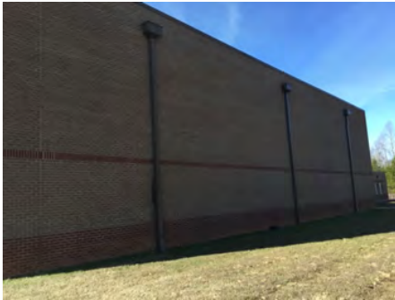
4). Northeast Elevation - Feb 13, 2017
