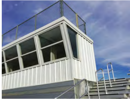
2). Southwest Elevation - Jan 24, 2017
