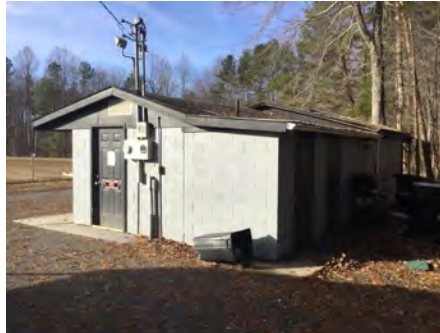
2). Northeast Elevation - Feb 10, 2017
