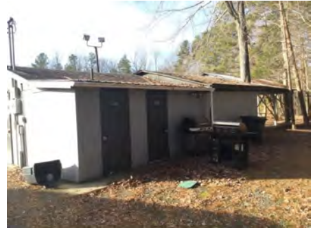
3). North Elevation - Feb 10, 2017
