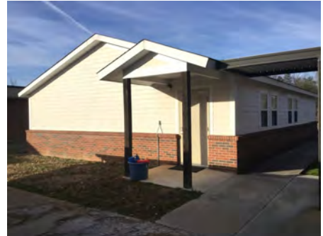
3). Northeast Elevation - Feb 10, 2017
