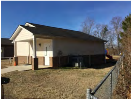
4). Northeast Elevation - Feb 13, 2017
