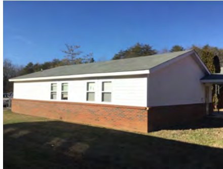
2). Southeast Elevation - Feb 10, 2017
