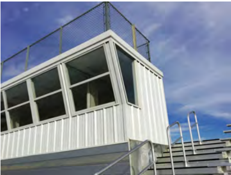
System: B2020 - Exterior Windows
