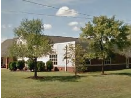
1). Southeast Elevation - Feb 14, 2017
