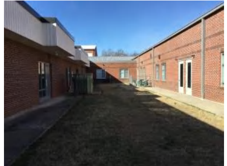
3). North Elevation - Feb 09, 2017
