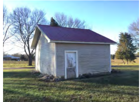
3). North Elevation - Feb 10, 2017
