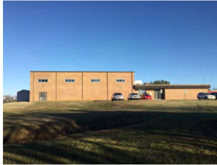
2). South Elevation - Feb 10, 2017
