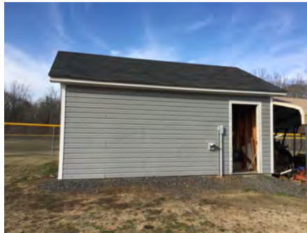
2). South Elevation - Feb 11, 2017
