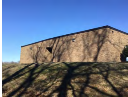
2). South Elevation - Feb 10, 2017
