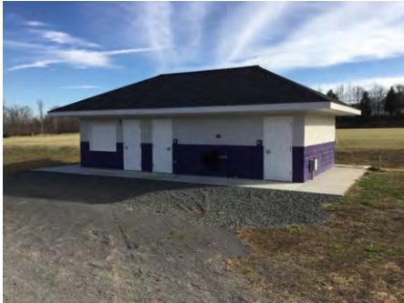
1). North Elevation - Feb 11, 2017
