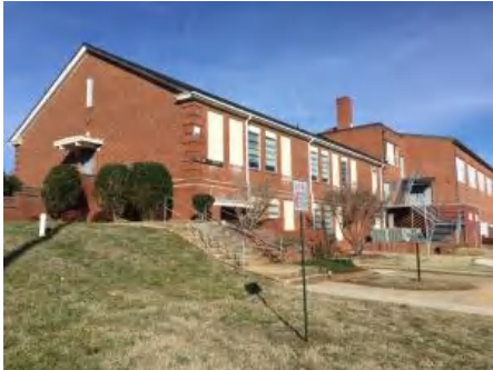
1). Southeast Elevation - Feb 09, 2017
