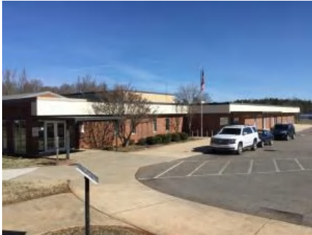
1). South Elevation - Feb 09, 2017
