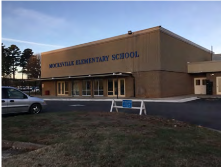
1). East Elevation - Mar 06, 2017
