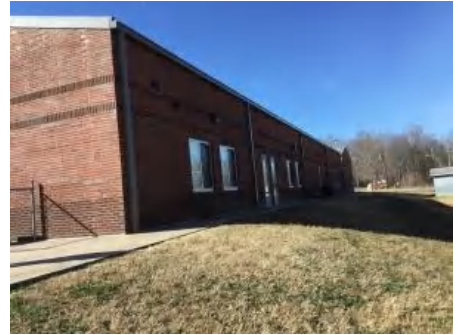
3). North Elevation - Feb 09, 2017
