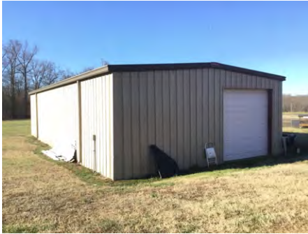
1). Northeast Elevation - Feb 10, 2017
