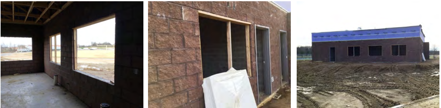
System: B2020 - Exterior Windows
