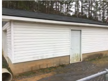
2). North Elevation - Jan 23, 2017
