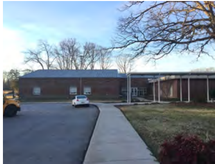
5). North Elevation - Feb 10, 2017
