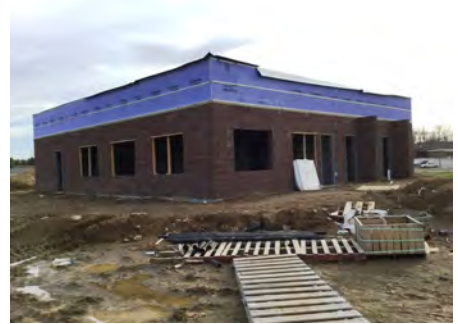
3). Northwest Elevation - Jan 24, 2017
