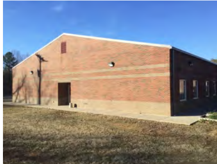
2). South Elevation - Feb 10, 2017
