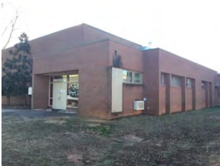
7). Northeast Elevation, Gym - Feb 10, 2017
