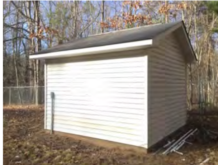
2). Northeast Elevation - Feb 10, 2017
