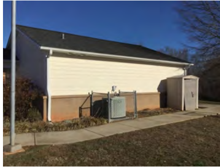
2). South Elevation - Feb 10, 2017
