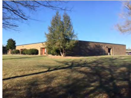
2). North Elevation - Feb 10, 2017
