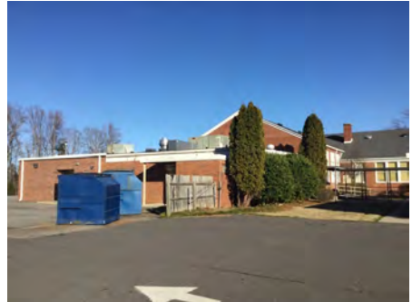
3). West Elevation, 1940 Bldg - Feb 10, 2017
