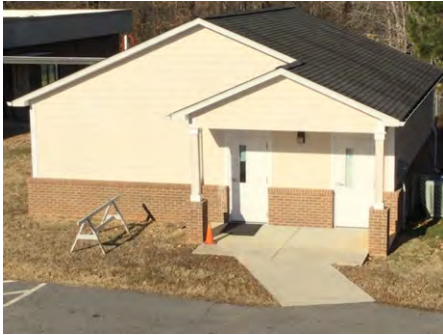
1). Southeast Elevation - Feb 13, 2017
