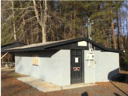
1). Southeast Elevation - Feb 10, 2017
