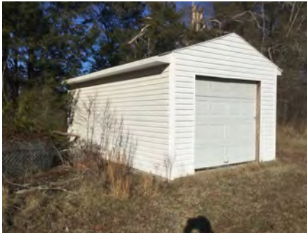
4). Southeast Elevation - Feb 10, 2017
