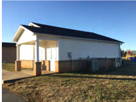
2). North Elevation - Feb 10, 2017
