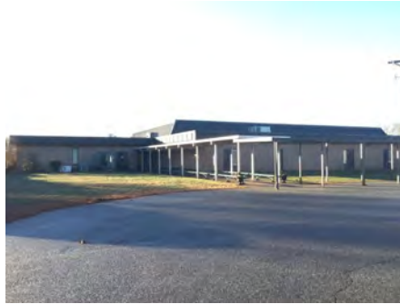
2). North Elevation - Feb 10, 2017
